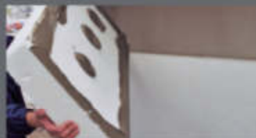
insulation board adhesive
